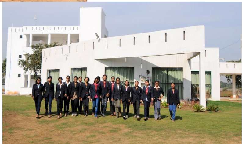
Modern academic infrastructure at the CPU Campus
